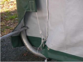
Door Turnbuckle Attached to Base Foot
