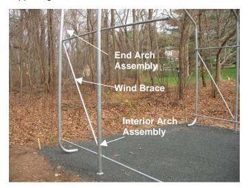
Begin the Top Ridge Cross Rail by placing a #7 Cross Rail FxF <u>underneath</u> the End Arch Top Crest Tube.
