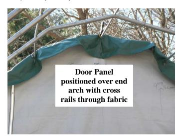
The rope channels should be located inside the unit, with the frame members passing through the pre-cut slots in the end panel/door. Replace and tighten the carriage bolts after putting the end panel into position.
