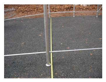
When all widths are adjusted properly, measure from diagonally from inside corner to inside corner. Adjust frame as necessary to bring frame into square. Failure to square frame of unit will result in poor cover fit and reduced strength and rigidity. If end or interior upright ends are placed on soft material that will not support weight, recess small patio blocks or bricks under leg ends. This will also allow better setting of frame before securing to ground.
