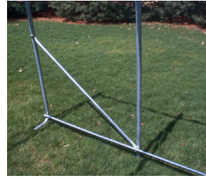
Structural wind brace on each side
